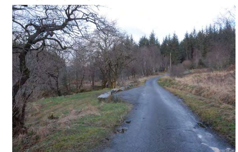
Layby with grass area protected by boulders
