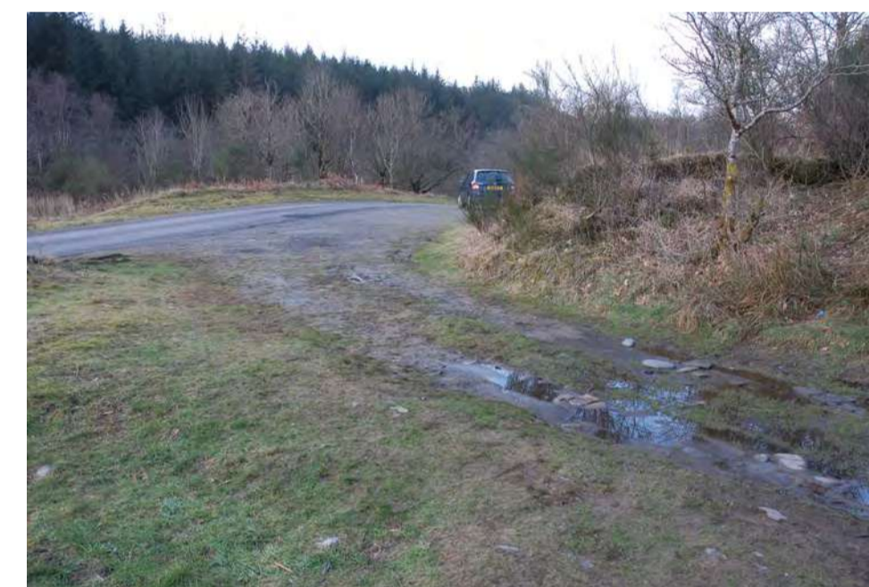
Damp area showing vehicle damage
